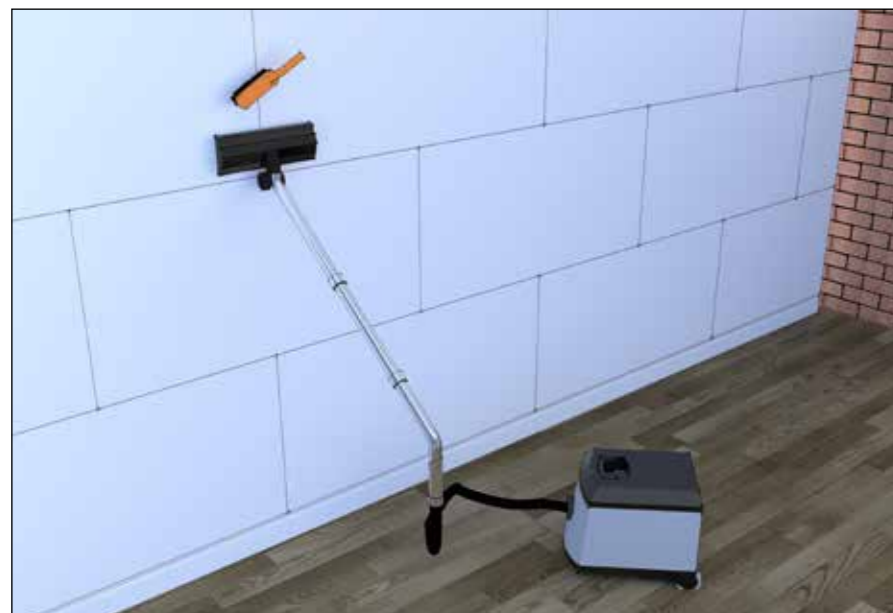
Fig. 7 Preparing Spacetherm WL surface for jointing
