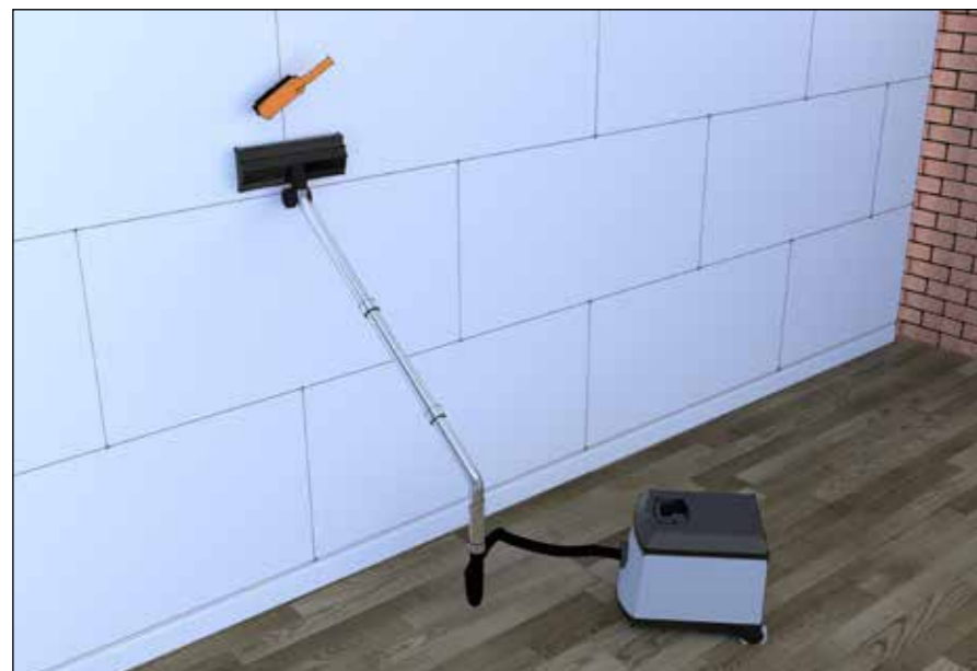
Fig. 7 Preparing Spacetherm WL surface for jointing
