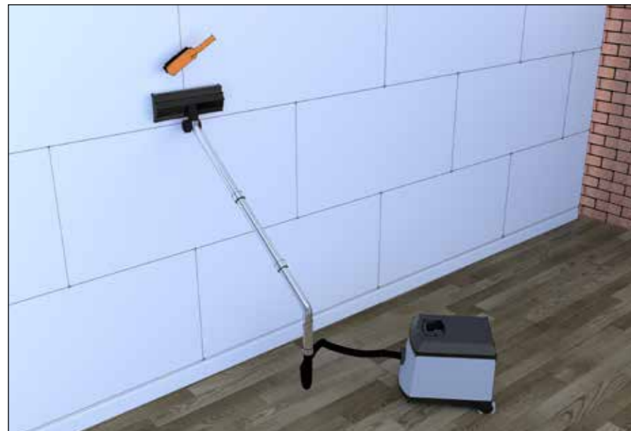
Fig. 7 Preparing Spacetherm WL surface for jointing
