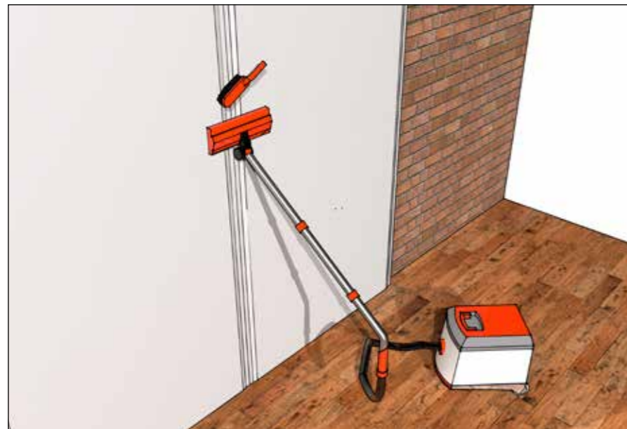
Fig. 7 Preparing Spacetherm Directfix Surface for Jointing
