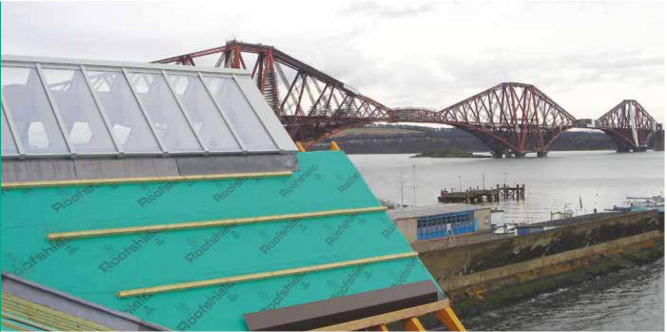
Forth Road Bridge
