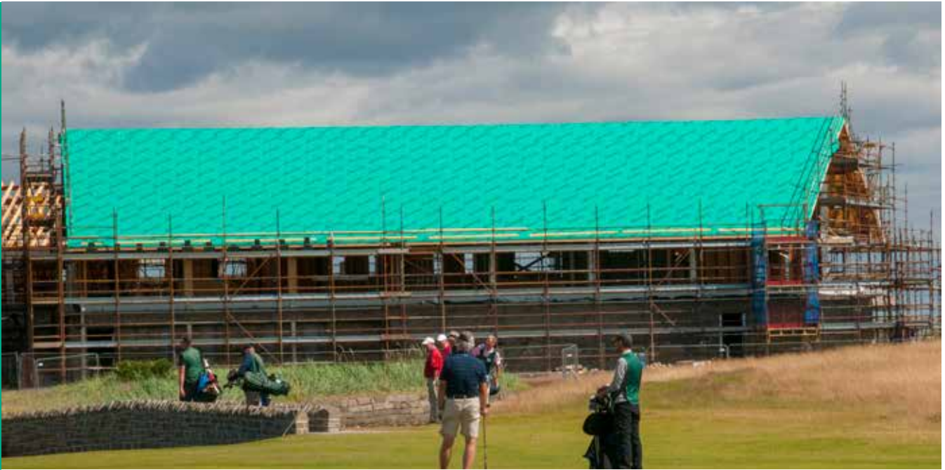
Carnoustie Golf Club Refurbishment
