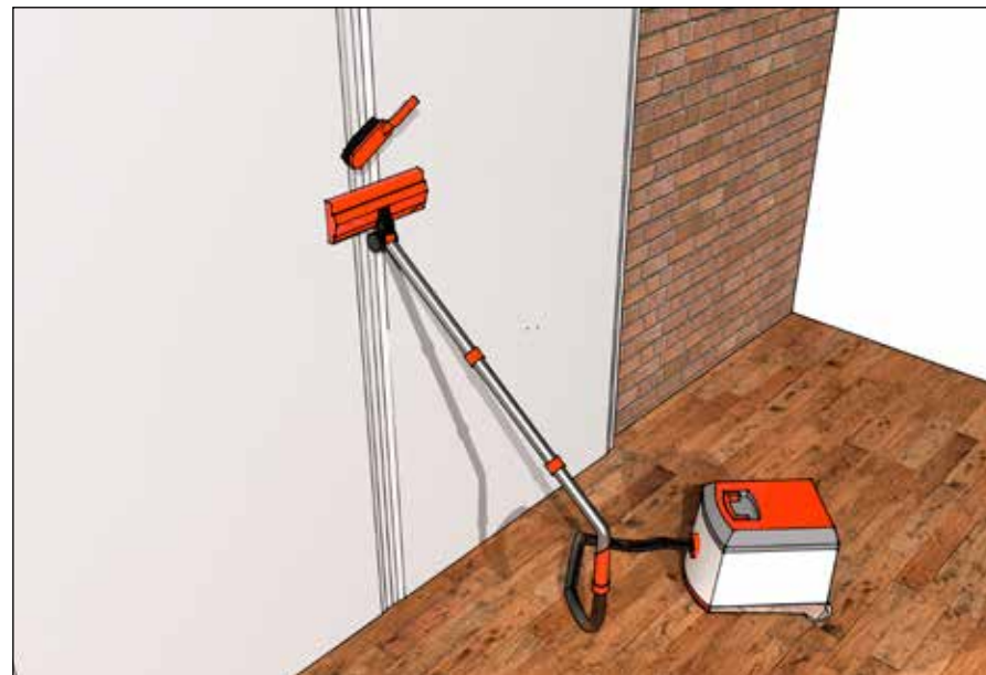
Fig. 7 Preparing Spacetherm Wallboard Surface for Jointing
