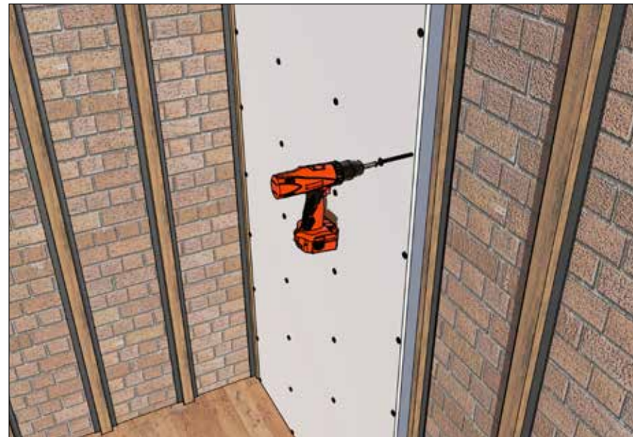
Fig. 4 Fixing Spacetherm Wallboard to Timber Straps
