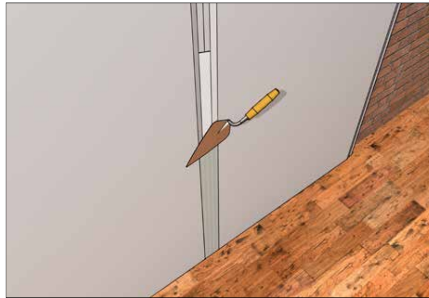
Fig. 8 Taping and Filling Joints in Spacetherm Wallboard
