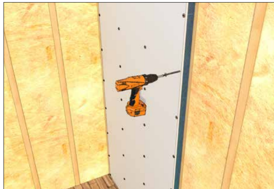
Fig. 4 Fixing Spacetherm Multi to Timber Straps
