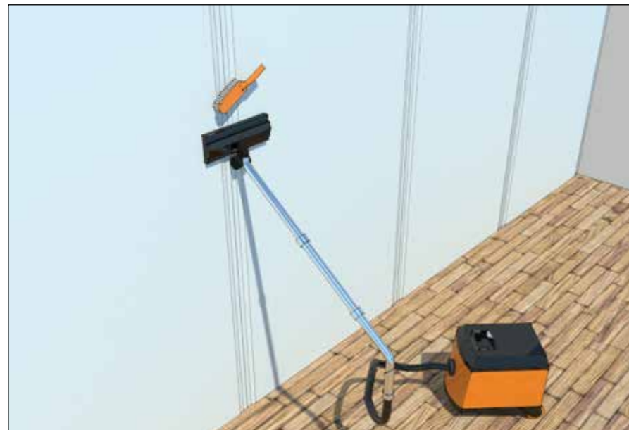
Fig. 7 Preparing Spacetherm Multi Surface for Jointing
