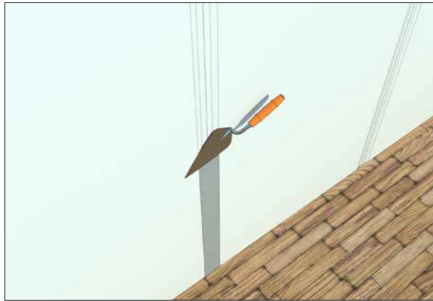
Fig. 8 Taping and Filling Joints in Spacetherm Multi
