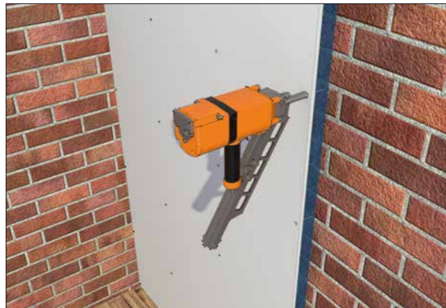
Fig. 4 Direct fixing Spacetherm Multi using nailgun
