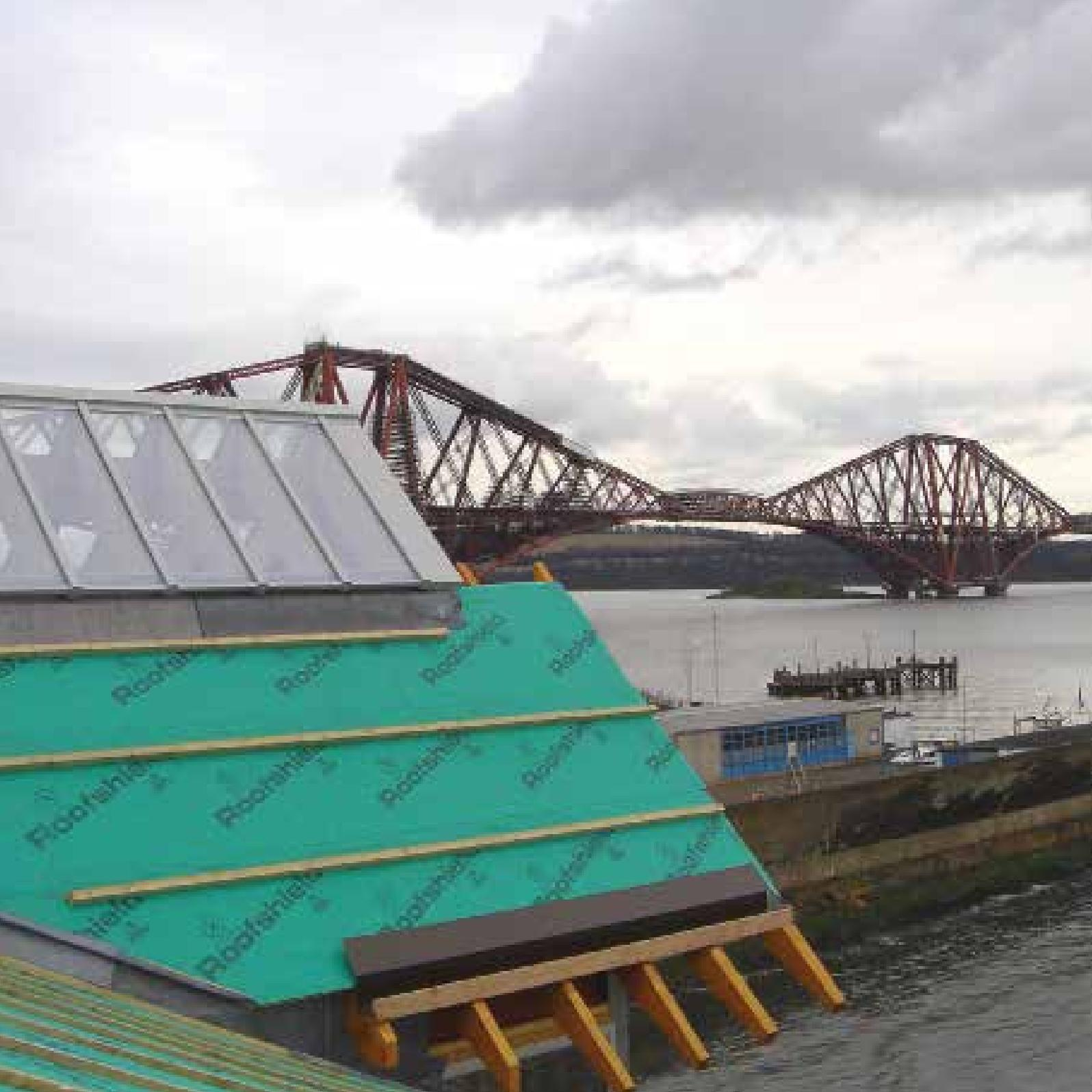
Roofshield is the highest performing breathable roofing membrane on the market, and has been independently tested for compliance with all UK wind zones as defined in the new BS 5534 standard.
