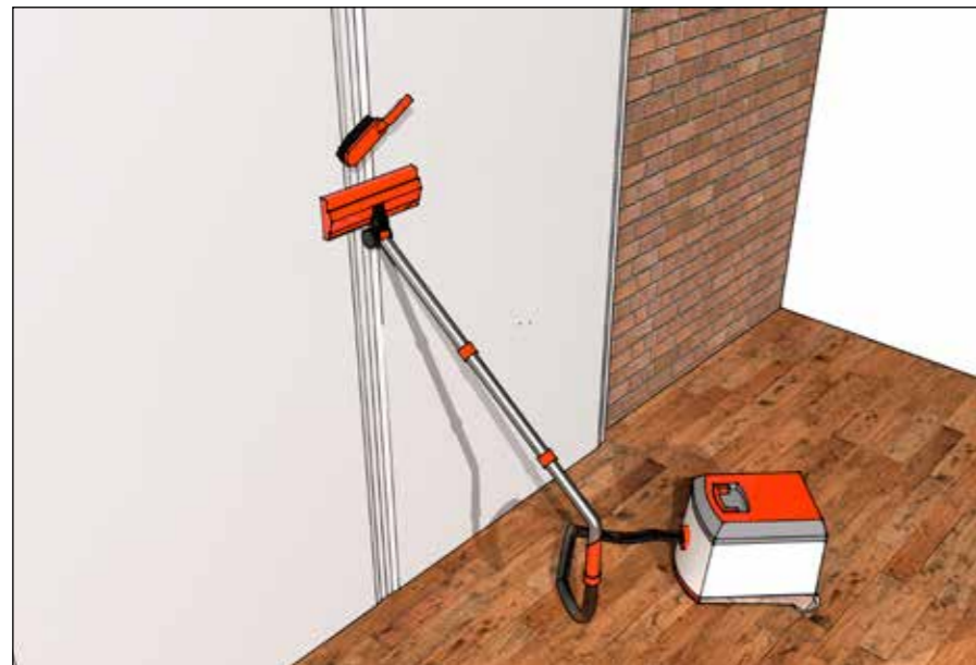
Fig. 7 Preparing Spacetherm Wallboard / A2 Wallboard Surface for Jointing
