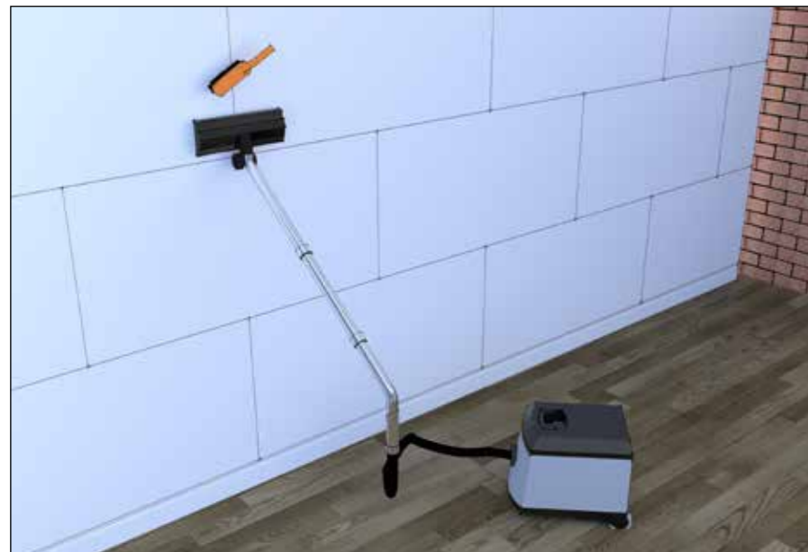
Fig. 7 Preparing Spacetherm WL surface for jointing
