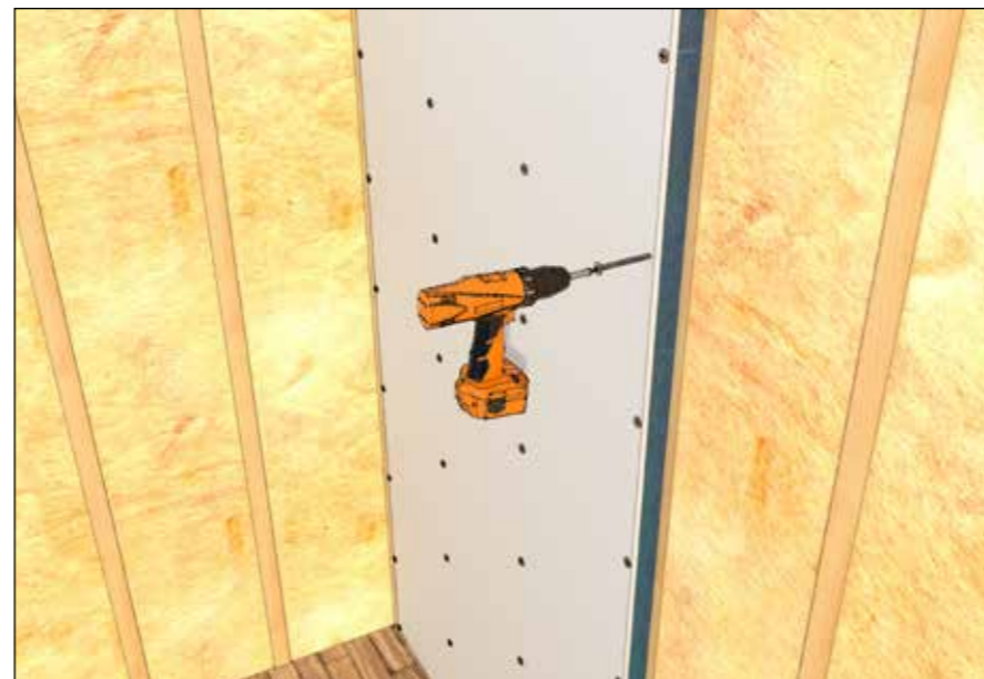
Fig. 4 Fixing Spacetherm Multi / A2 Multi to Timber Straps
