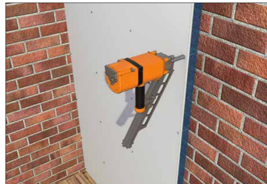
Fig. 4 Direct fixing Spacetherm Multi using nailgun
