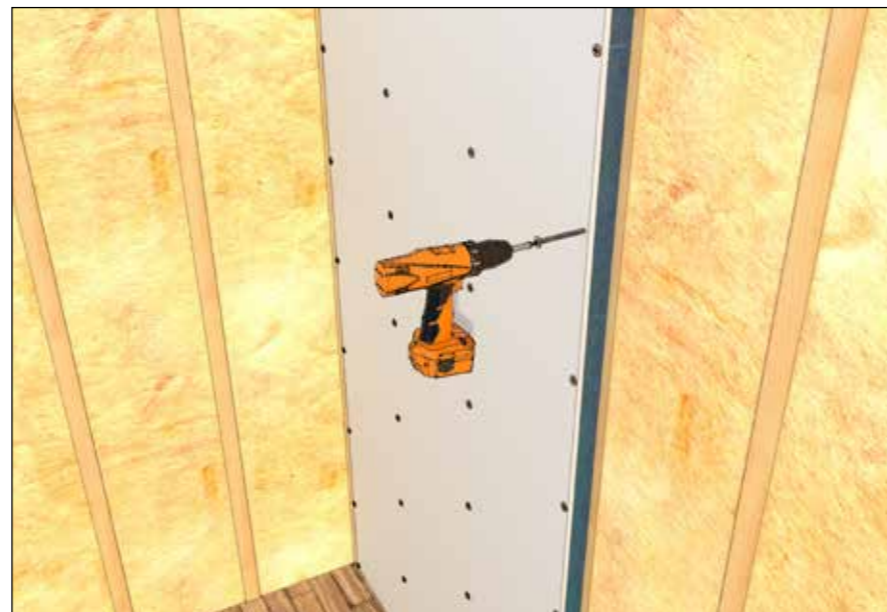
Fig. 4 Fixing Spacetherm Multi to Timber Straps
