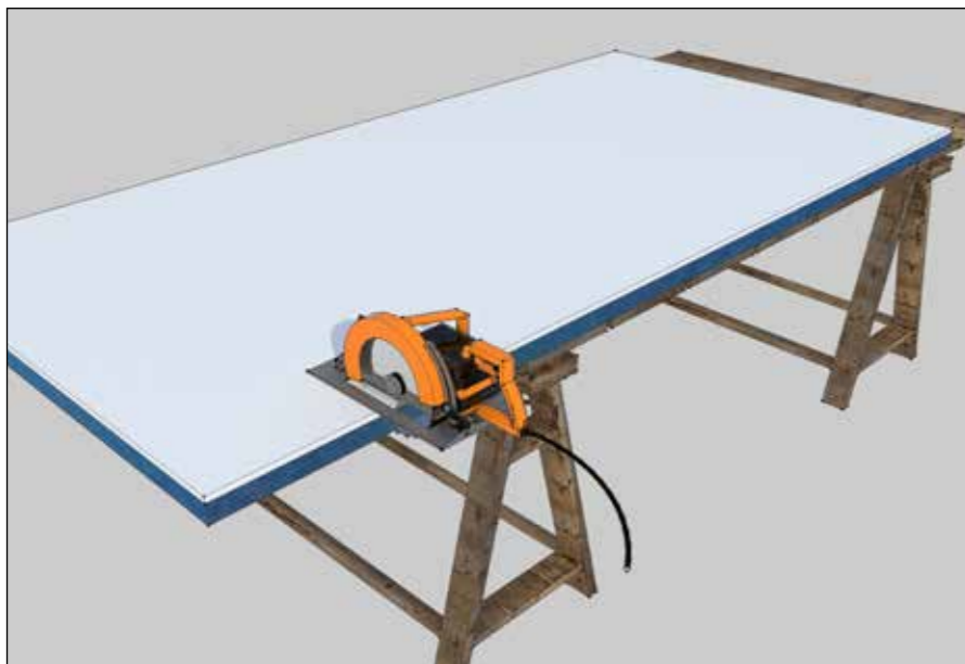
Fig. 2 Cutting Spacetherm Multi Boards
