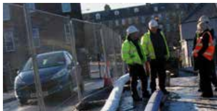
Shallow water piping process
