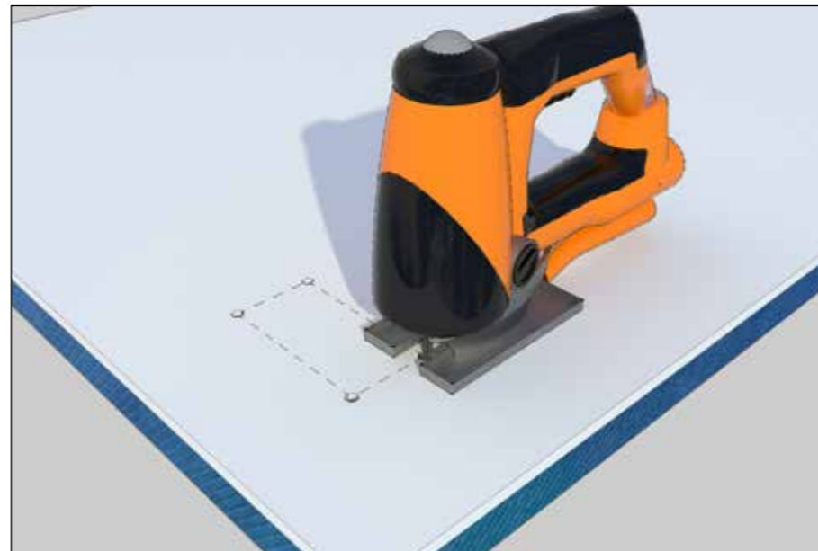
Fig. 3 Making cut-outs in Spacetherm Multi
