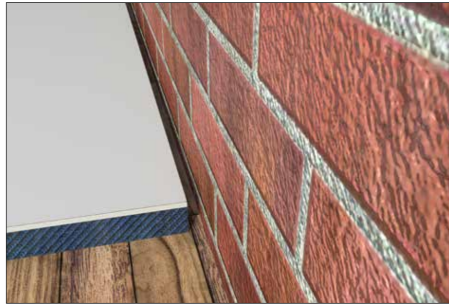
Fig. 6 Expansion gap at perimeter of Spacetherm Multi
